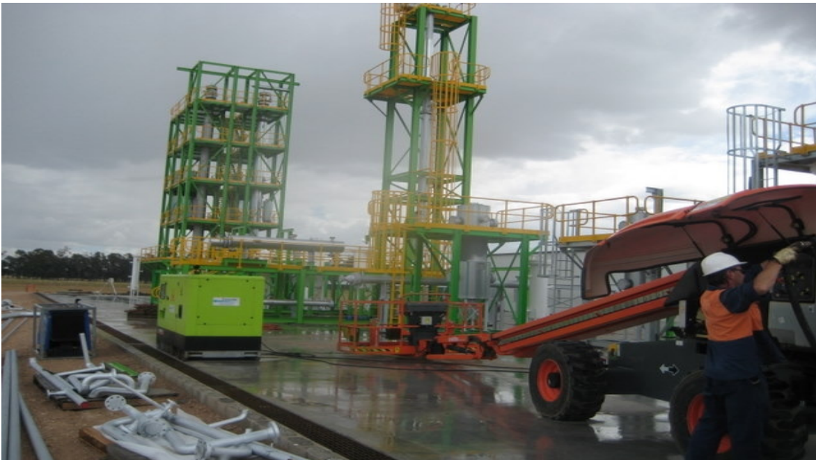
FIGURE 2: LINC ENERGY SITE VISIT – LNC'S GTL FACILITY
